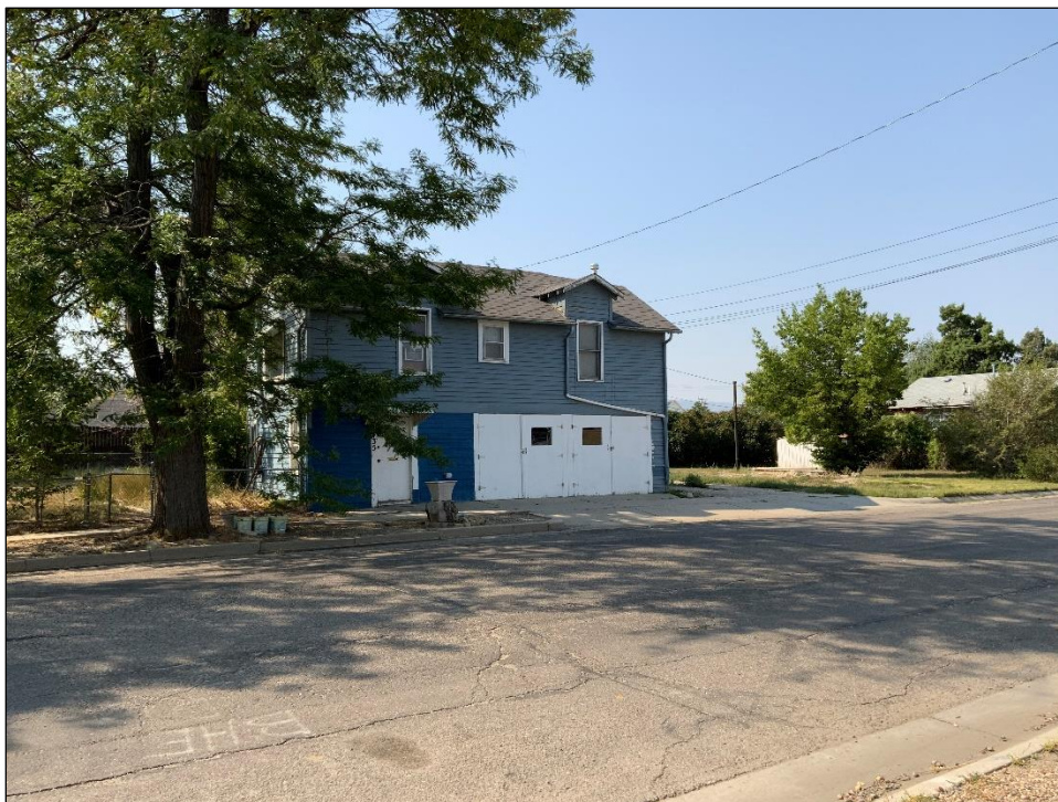
Photo 23. Overview image of the House of Ruth, view south-southwest.
