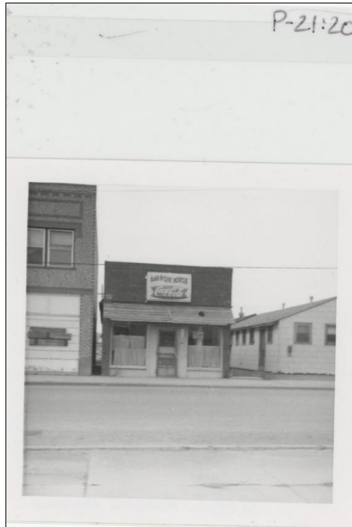
Photo 3. Representative image of a false front store (center) as well as brick construction (left) and tarpaper/shingling (right). Image courtesy of the Western History Center.
