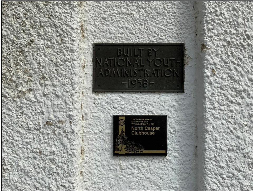
Photo 9. Close-up image of the plaques on the north wall of the building.
