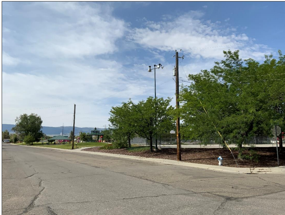
Photo 7. Overview of the northern portion of the Mathew Campfield Park, view southwest.
