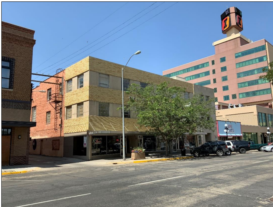
Photo 15. Overview image of the Odd Fellow’s building in downtown Casper, view northwest.
